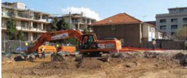
Camperdown: Earthworks commence
